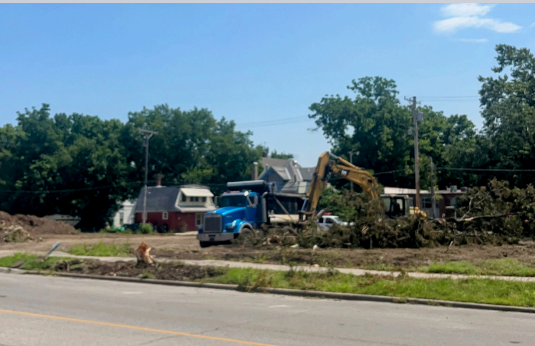
Construction underway on developer Krsnich's New Hampshire project
